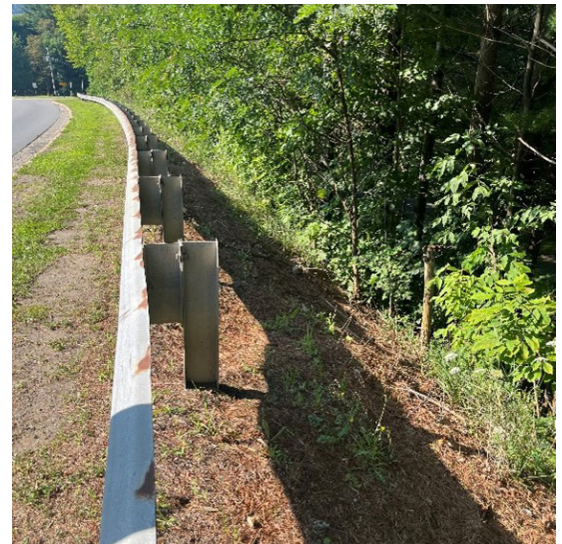
Steep terrain behind guardrail along South Jefferson Avenue
