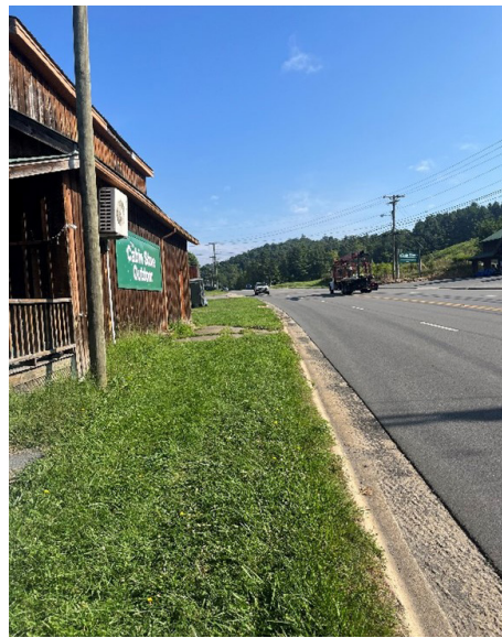
Existing building located close to roadway along South Jefferson Avenue
