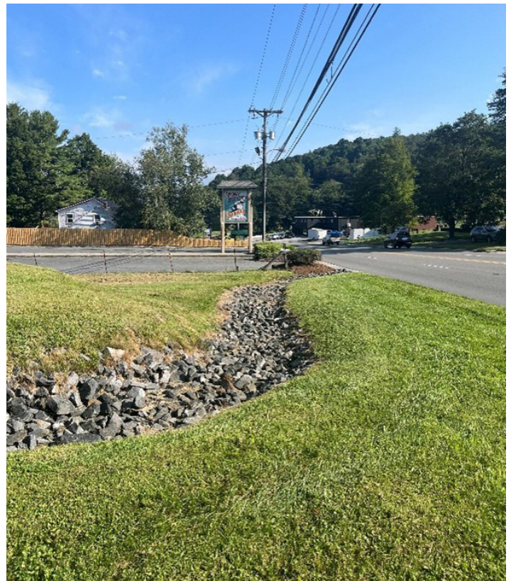
Retention pond and outlet ditch into roadway along South Jefferson Avenue
